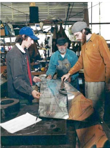
HSU Students using a Beverly shear to cut aluminum sheets into triangular facets.
